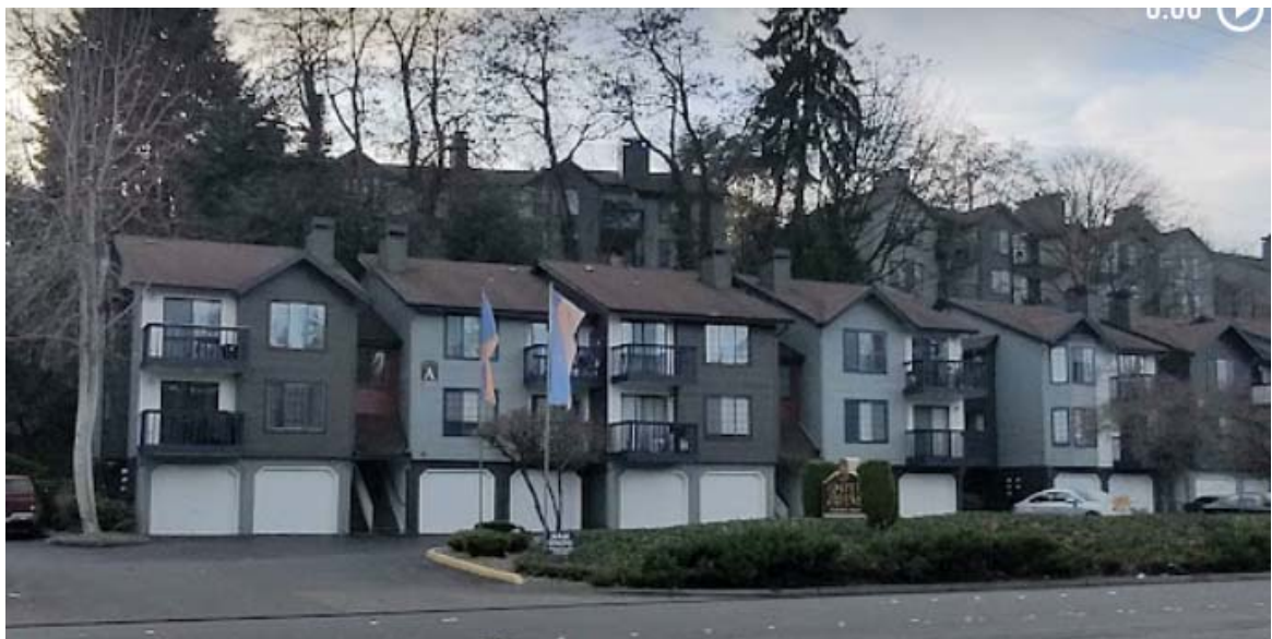
Figure 13: Interurban Ave S Residential Development (north of project site)
