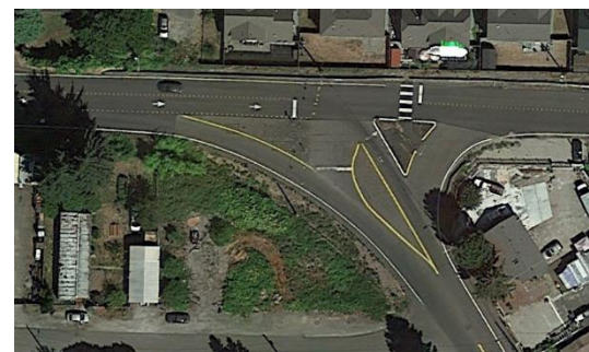
S 124th Street/50th Place S intersection
