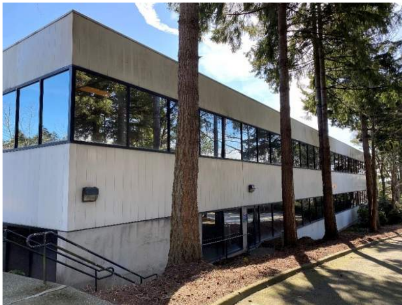
Figure 3.2-1. 6300 Building, West Exterior.
