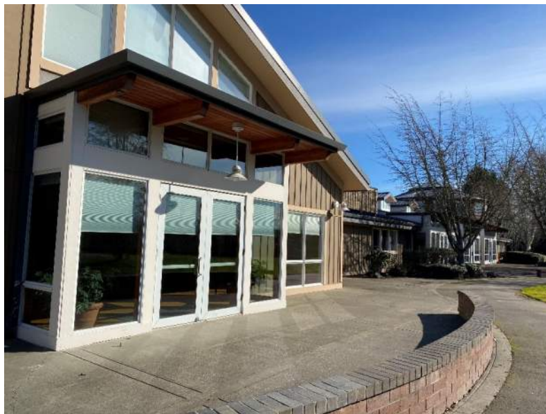
Figure 3.3-2. Community Center, West Exterior.
