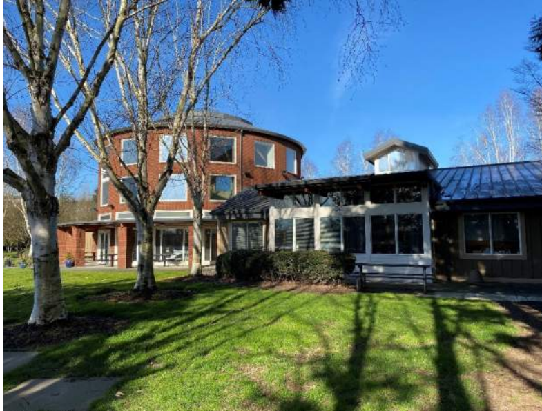
Figure 3.3-1. Community Center, Southeast Exterior.
