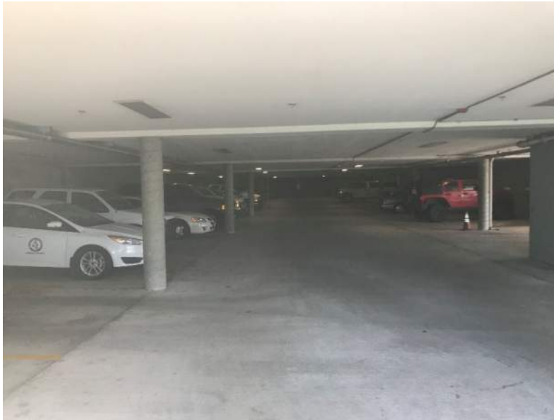
Figure 3.2-2. 6300 Building, Parking Level.
