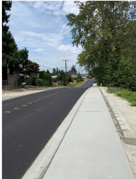
Macadam Road S. looking north after construction
