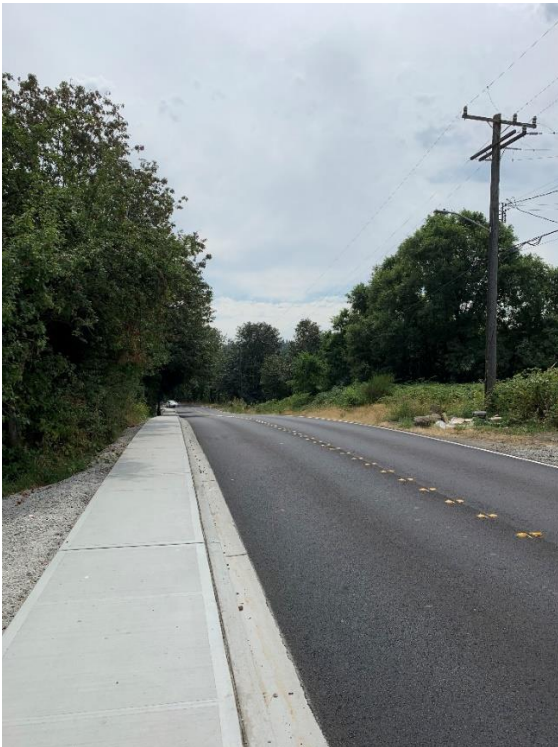
Macadam Road S. looking south after construction
