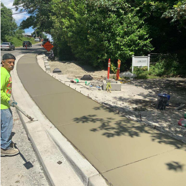
Macadam Road S. sidewalks during construction
