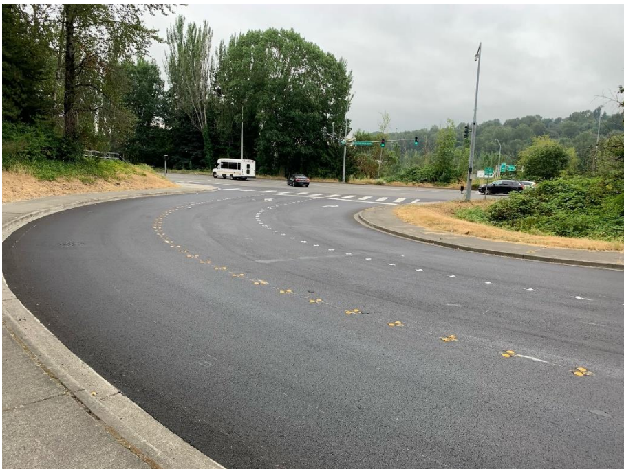
Macadam Road S./Southcenter Blvd. intersection after construction
