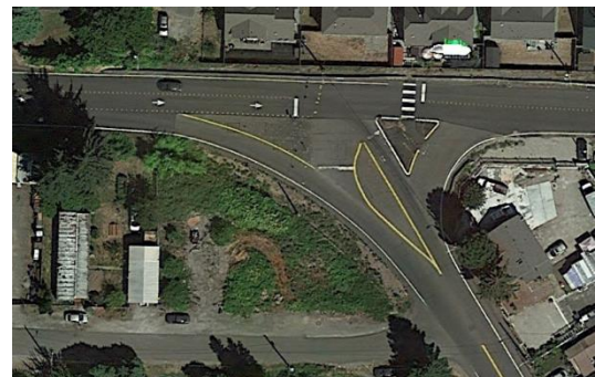
S 124th Street/50th Place S intersection
