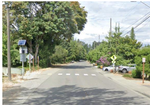
42nd Avenue S at S 119th Street (looking north)
