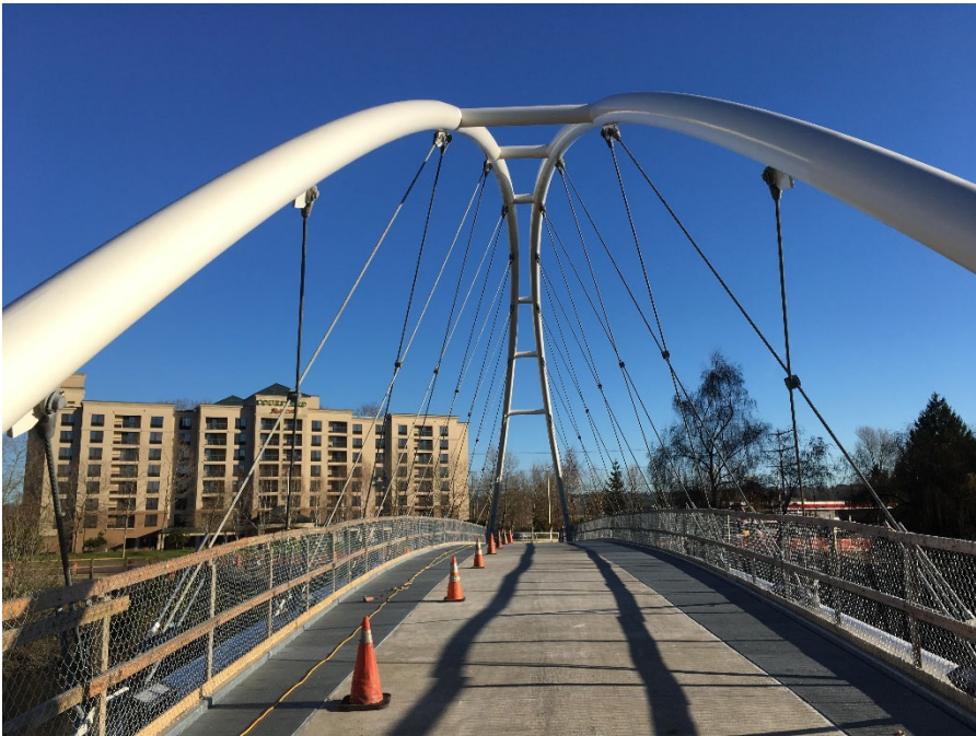
Tukwila Urban Center Pedestrian Bridge
