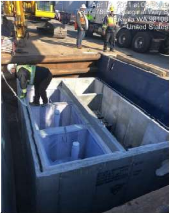
Stormwater media filter unit installation
