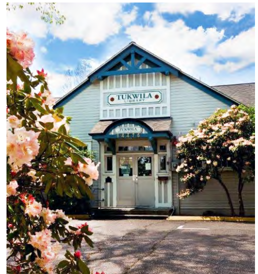
Original Tukwila City Hall Building
