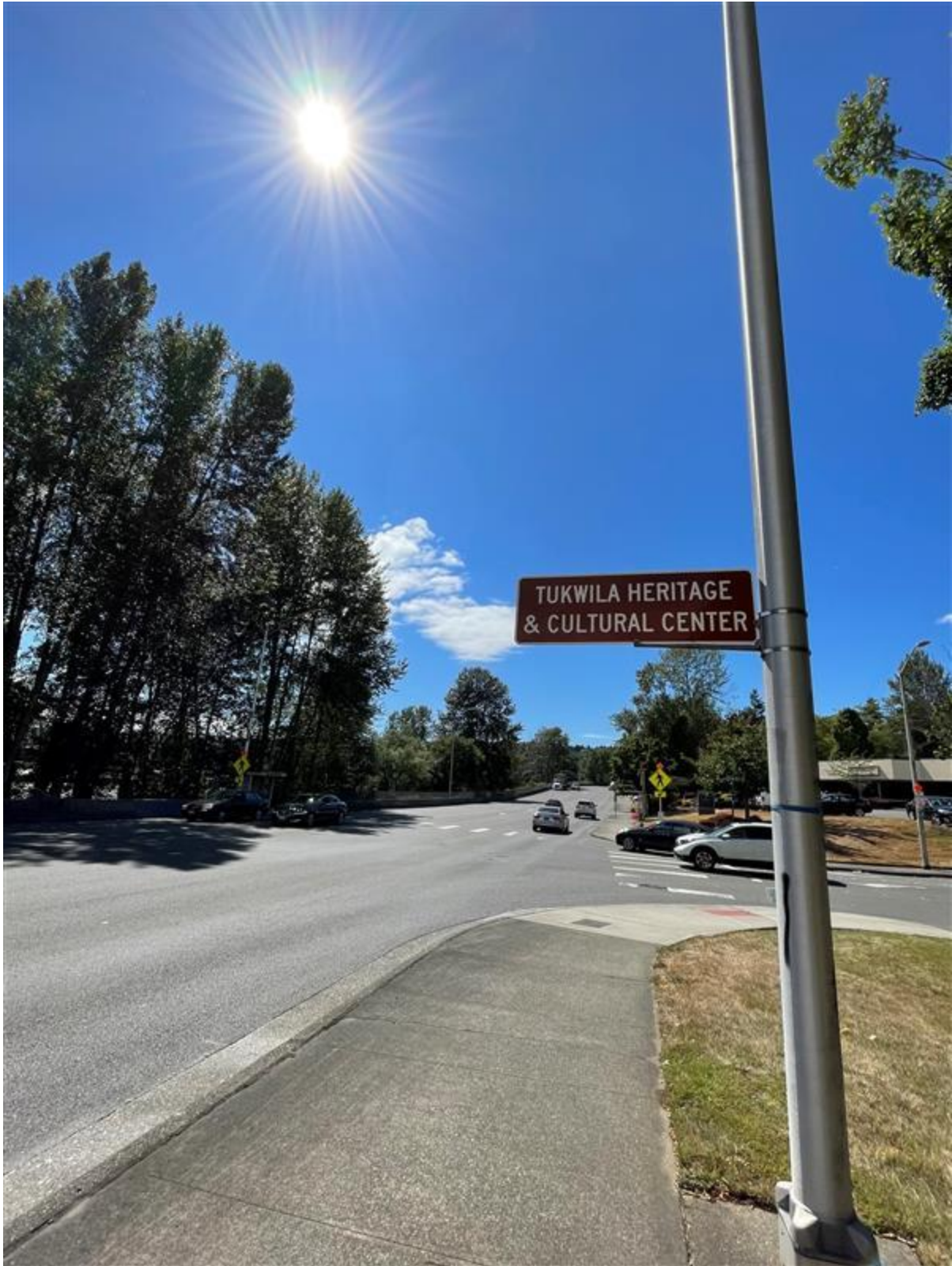
Southcenter Blvd/65 th Ave S Signal Facing West
