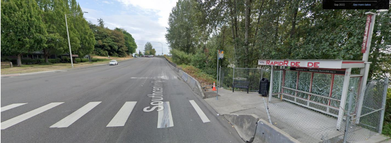
Southcenter Blvd/65 th Ave S Signal Facing East at the Bus Stop
