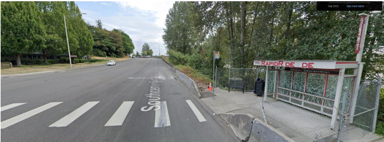
Southcenter Blvd/65 th Ave S Signal Facing East at the Bus Stop
