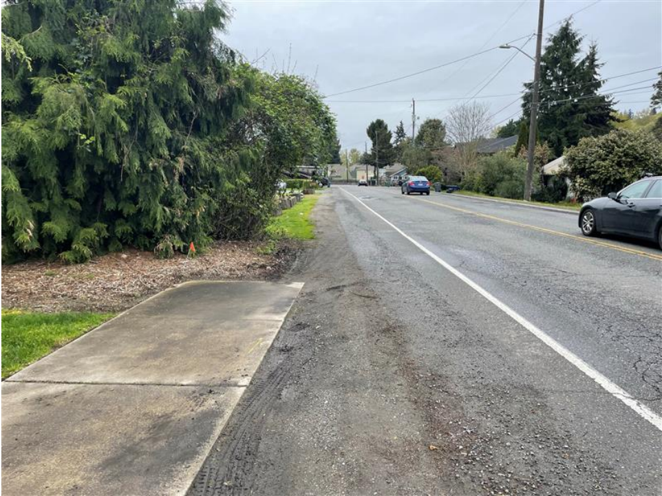
Cracking on roadway, missing RPMs, and faded paint on 50 th PI facing North
