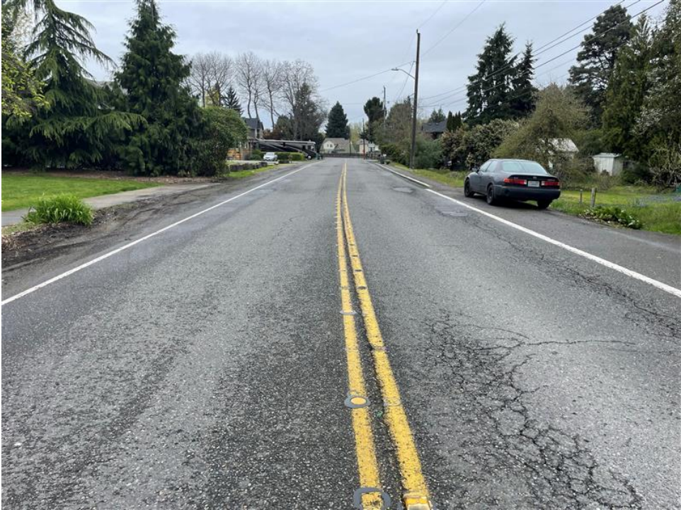
Cracking on roadway, missing RPMs, and faded paint on 50 th PI facing North
