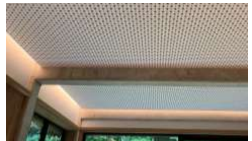
Ceiling installed acoustic panels in a common area. Photo courtesy of Schemata Workshop.
