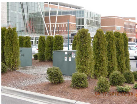
Figure 31 Using evergreen landscaping to screen utilities
