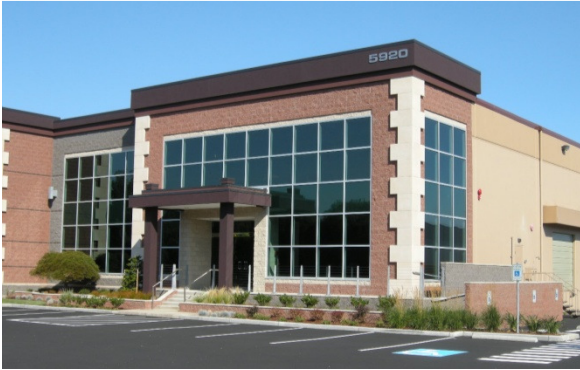
Warehouse redevelopment on S.180 th St
