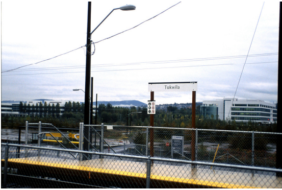
Photo 8. Temporary Tukwila Longacres Station
