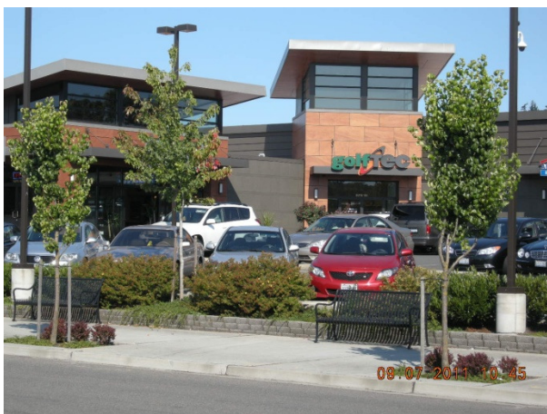
405 Baker Blvd. – redevelopment of warehouse with public frontage improvements
