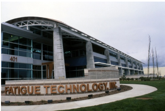
30. Existing light industrial/warehouse
