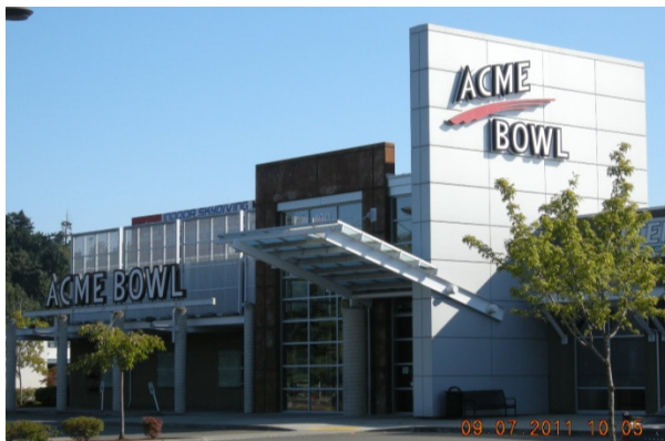
Acme Bowl – redevelopment of warehouse
