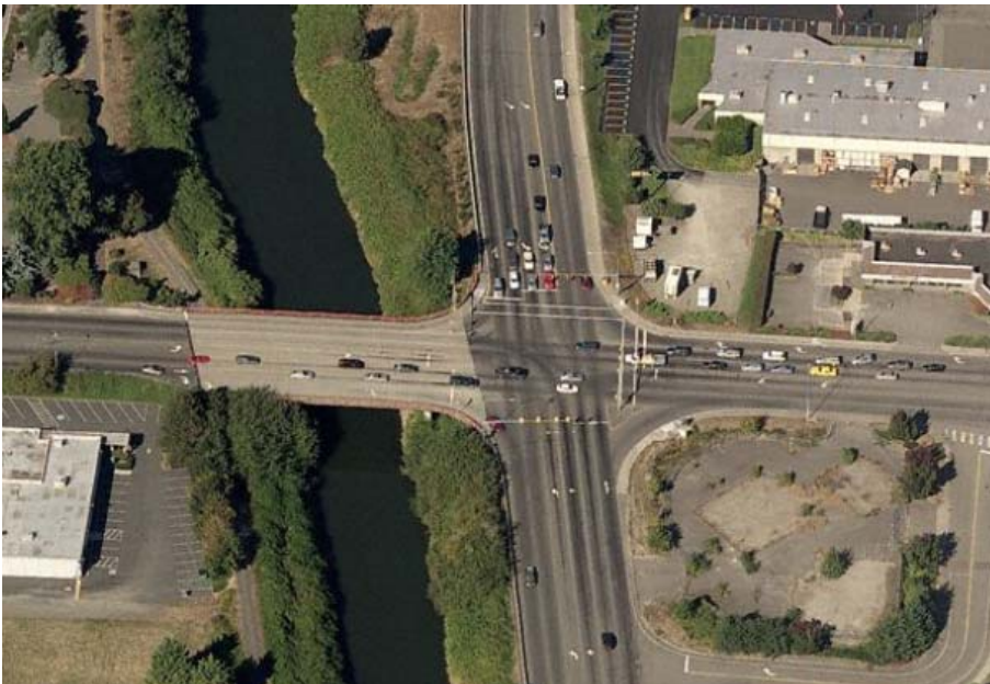
Aerial photo of the S 180th Street/West Valley Highway intersection.
