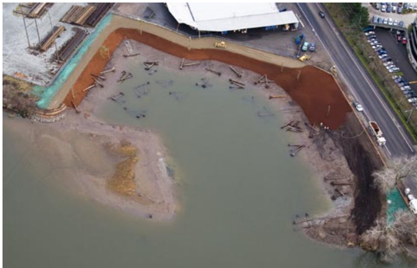
Aerial View of North Winds Weir Off-Channel Habitat (photo courtesy of WRIA 9)
