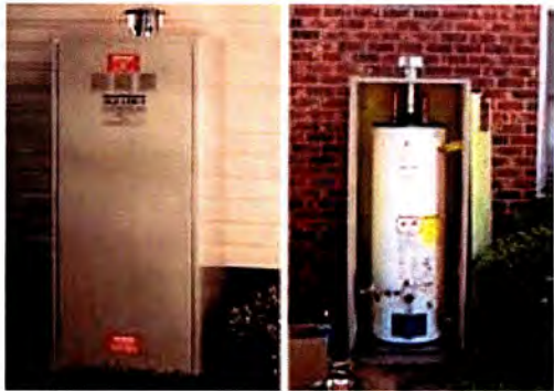
Sample of an enclosure on a concrete pad. Can be metal or wood. Roof must be weatherproof.
