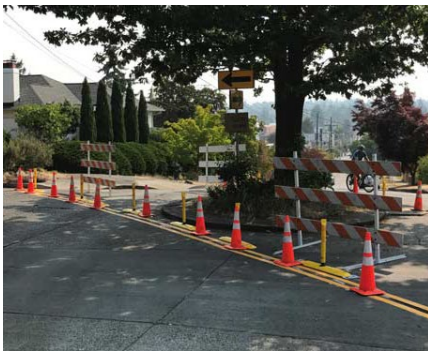
Temporary traffic diverters in Seattle. Source: Chris Sullivan/KIRO Radio 11
