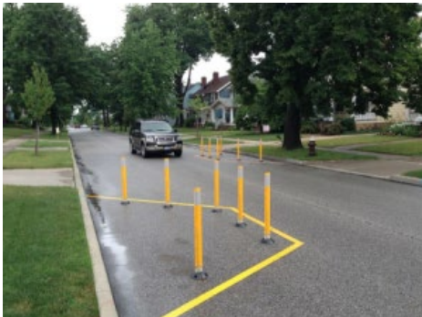
Temporary chicanes in Bend, OR. Source: Bend Bikes 3
