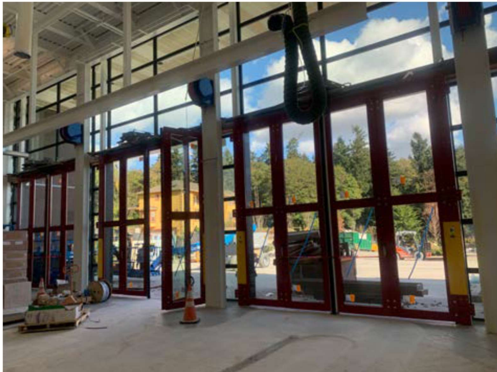
Four Fold Door Installation
