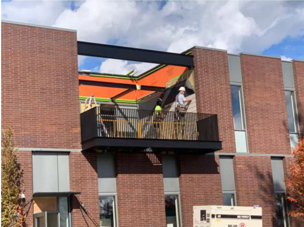
Fiber Cement Planks Installed At Deck
