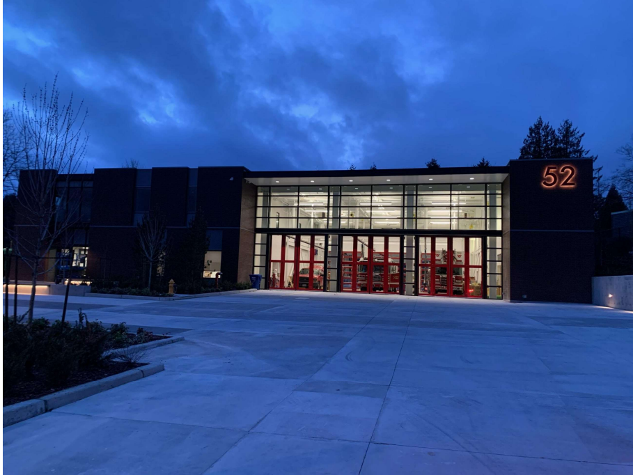
Exterior Fire Station 52 Signage Installed
