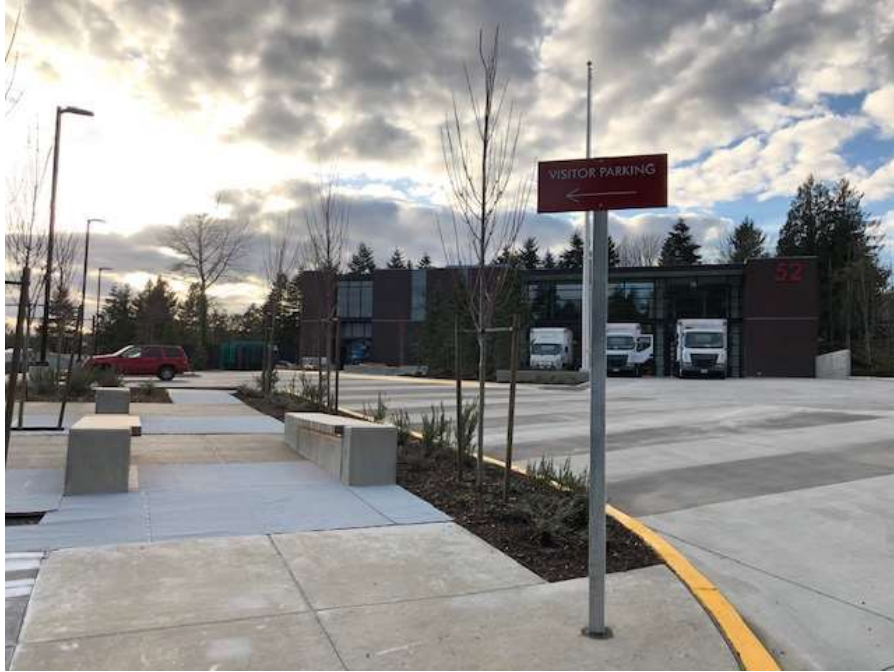
View looking toward fire station apparatus bay
