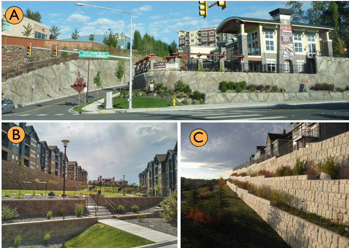
Figure 2.8.B Appropriate retaining wall terracing.
