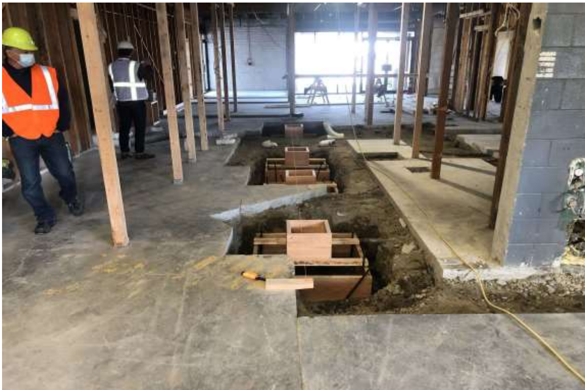
OFFICE AREA FOOTING FORMS IN PLACE
