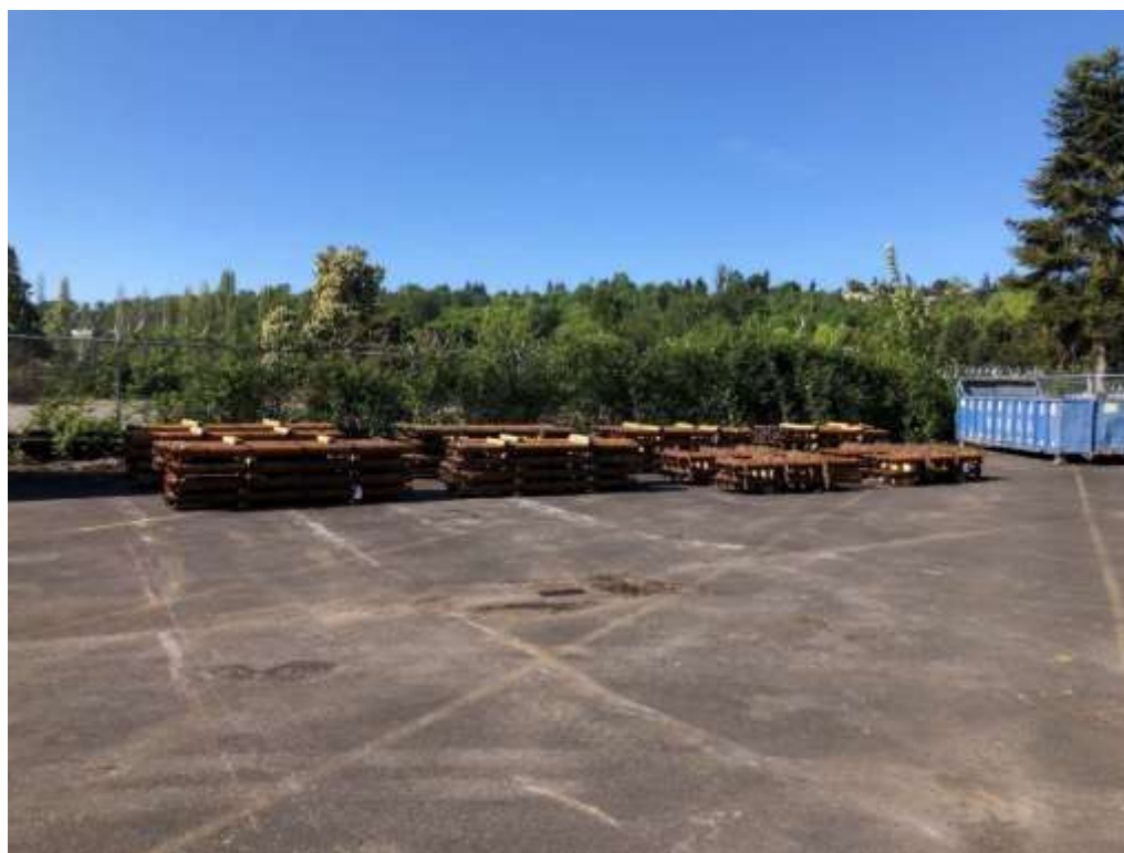
HELICAL PILES ON SIT
