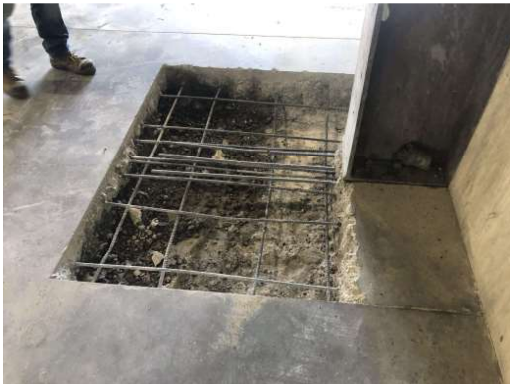
REINFORCING DISCOVERY IN EASTERN BUILDING FOOTINGS
