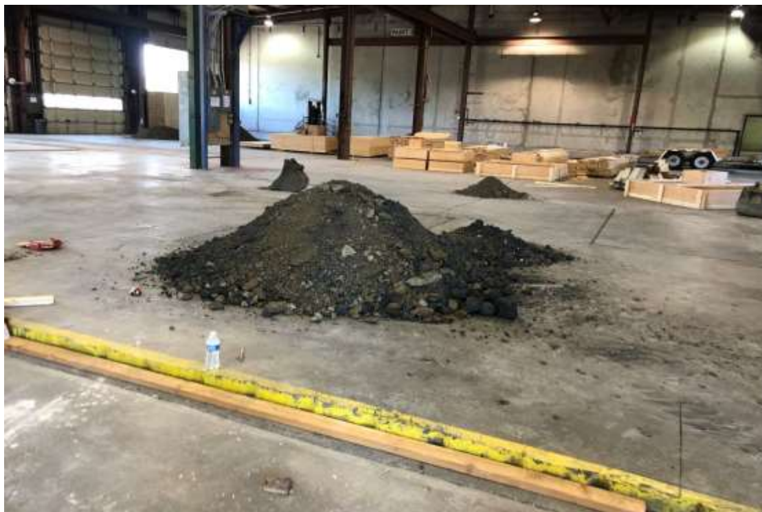
EXCAVATED CONTAMINATED SOILS – AWAITING TESTING RESULTS
