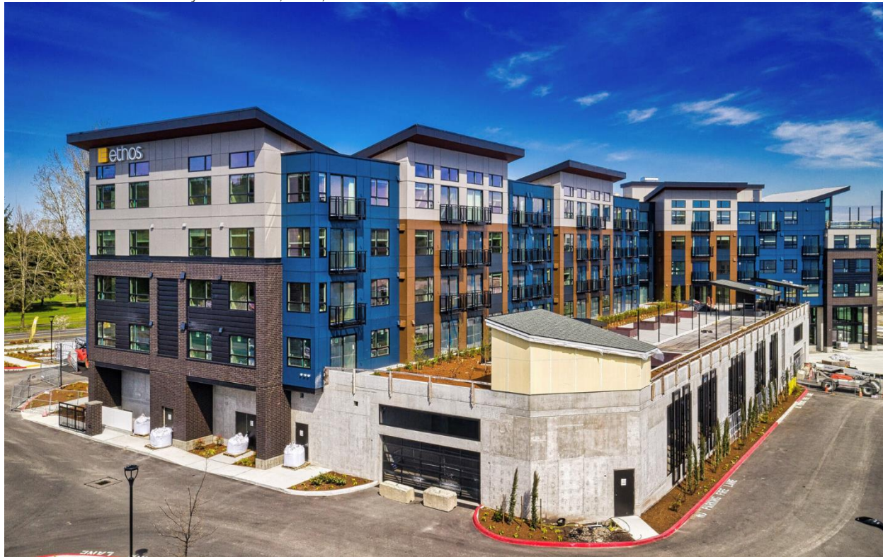
Figure 34. Example of a 4-over-2 Podium Development with Structured Parking
