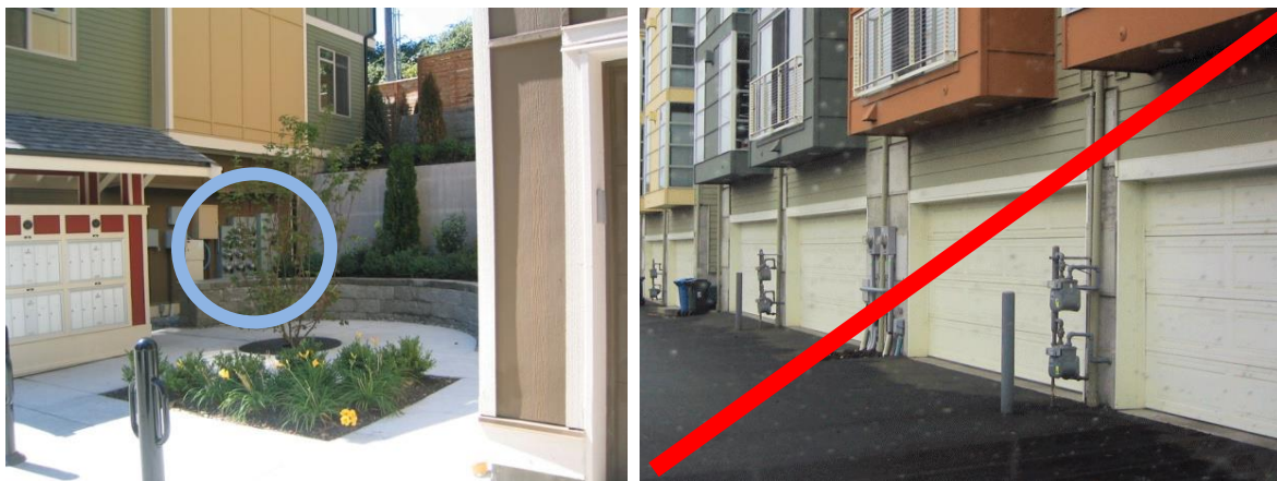
Utility meter location and screening - good and bad examples.
