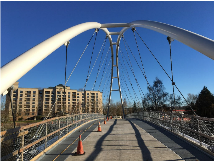
Tukwila Urban Center Pedestrian Bridge
