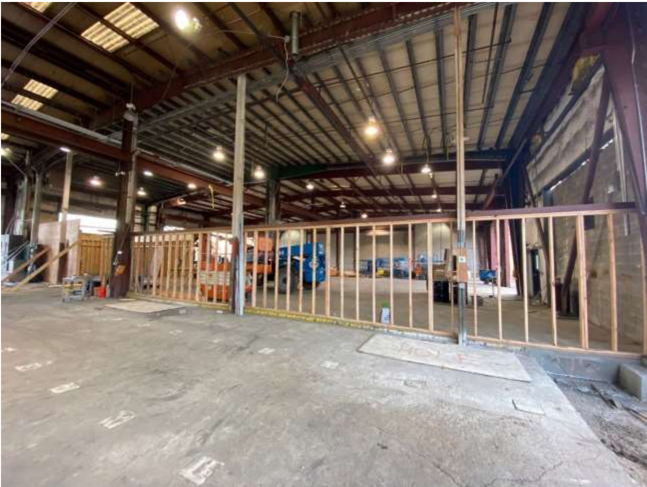
Framing in West Building
