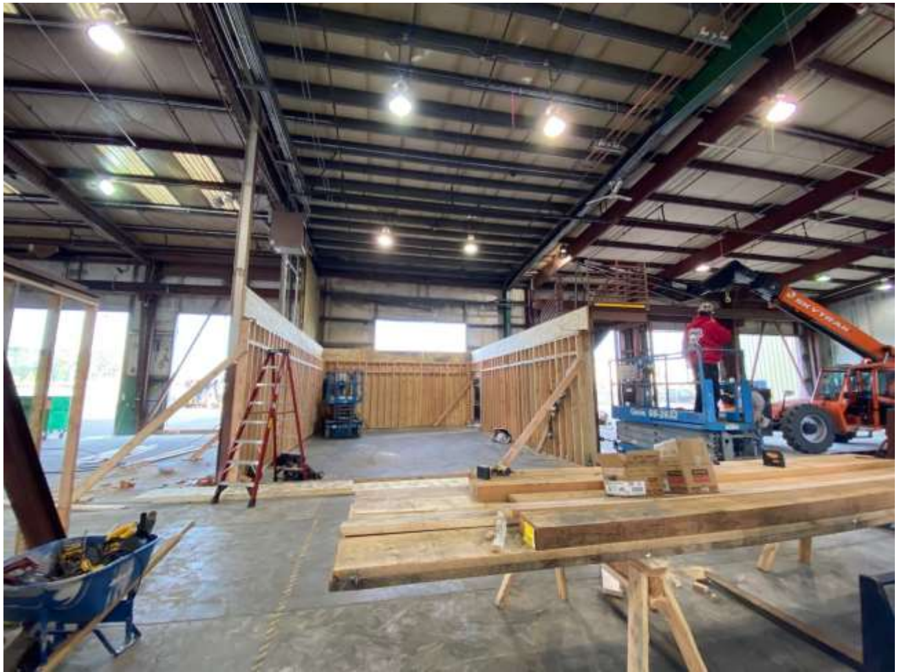
Framing Fleet Offices
