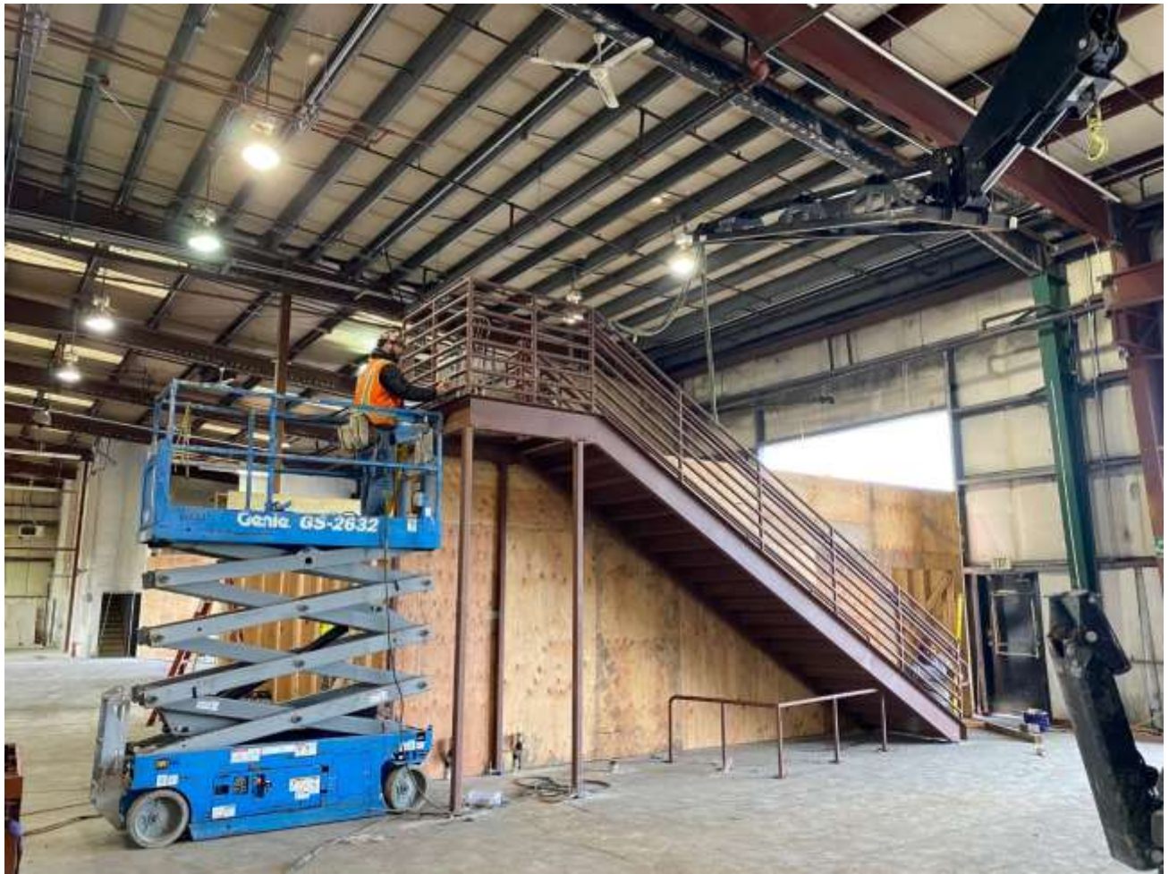
Installing Upper Level Storage Staircase
