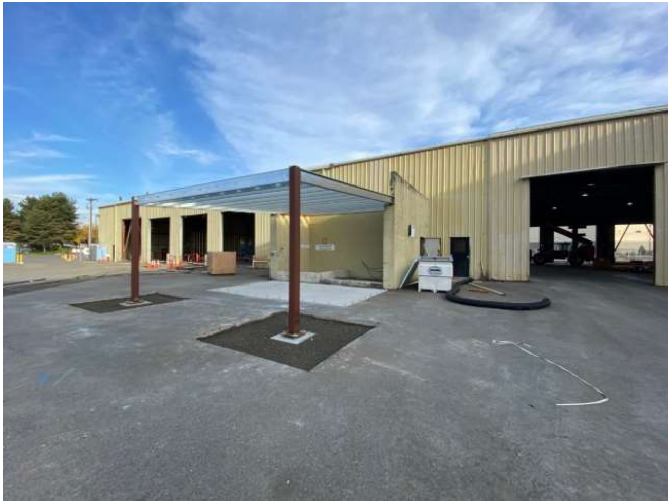
South Side of Building – Shed Roof
